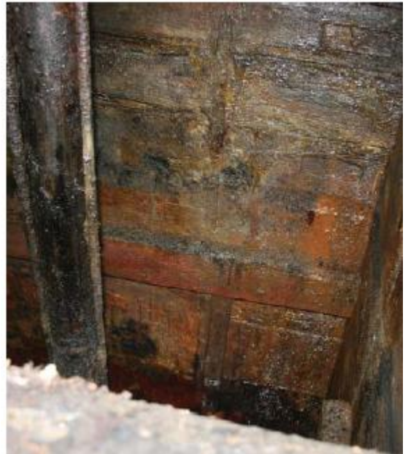
Timber lined shaft
