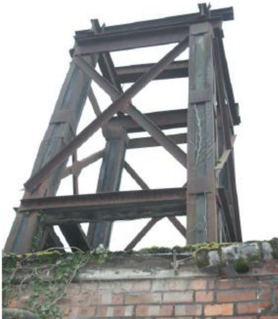
Timber head gantry
